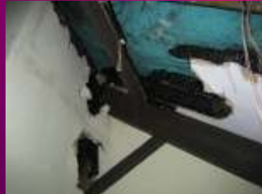
Result of an unenclosed downlighter fire
