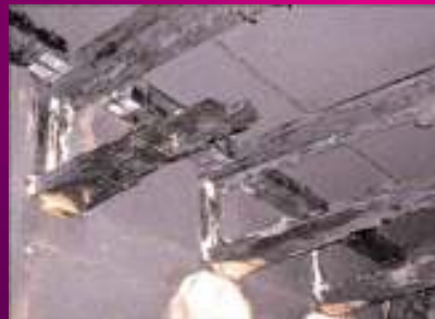
Result of an eight minute fire on lightweight joists
